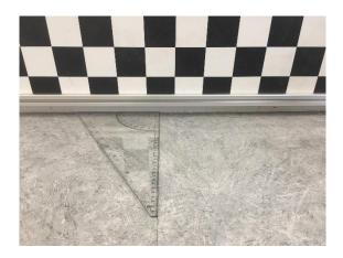
Finding a line perpendicular to the wall
